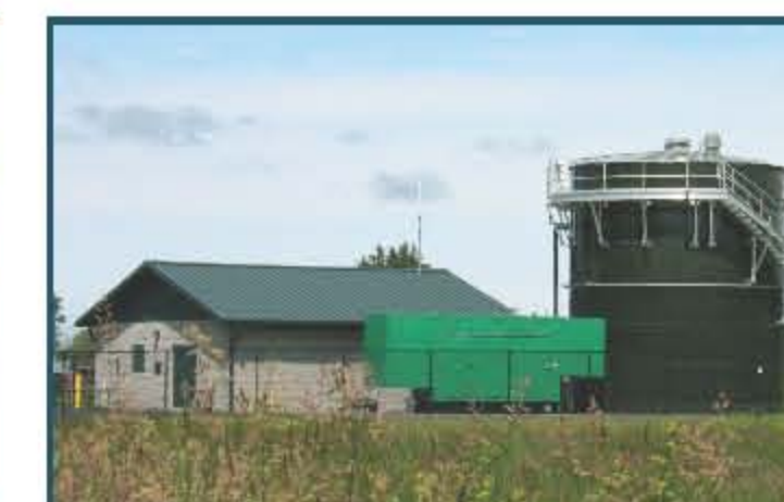
8. The vacuum station building is designed to fit the characteristics of the surroundings
