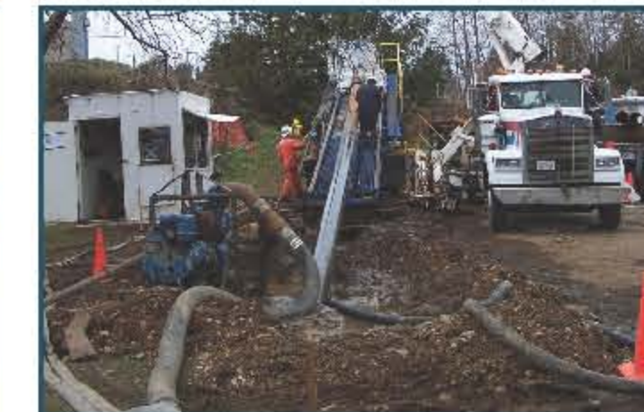
4. Horizontal directional drilling of force main under Youngs Bay
