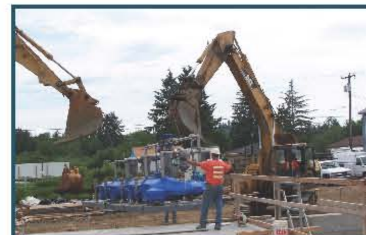
6. The skid-mounted equipment is placed into the vacuum station building
