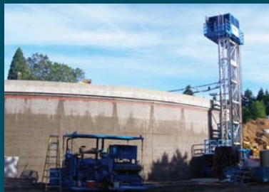
State-of-the-art Wire Wrap Concrete Prestressing
